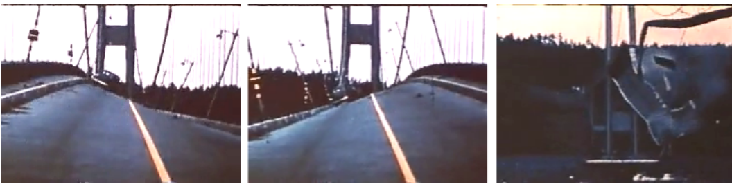
Figure 1.2: Collapse of the Tacoma Narrows Bridge (1940).
