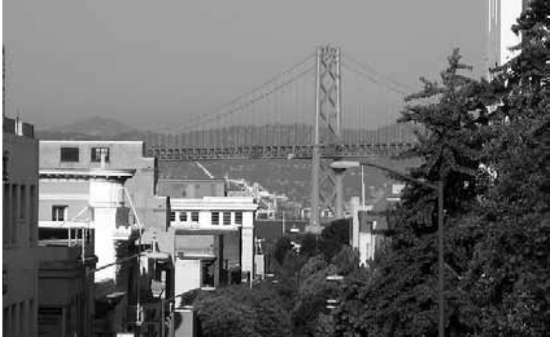
San Francisco Oakland Bay Bridge.
