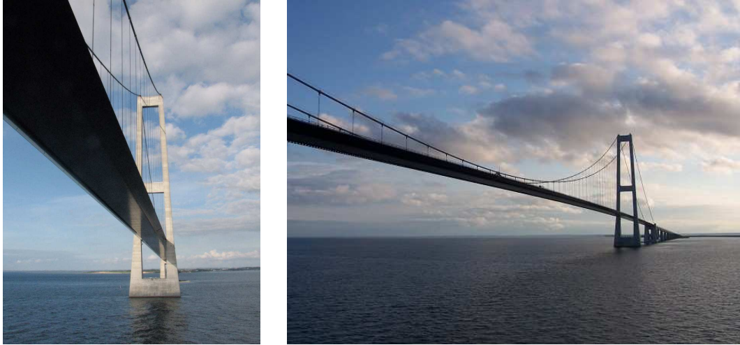
Figure 3.3: Great Belt East suspension bridge.
